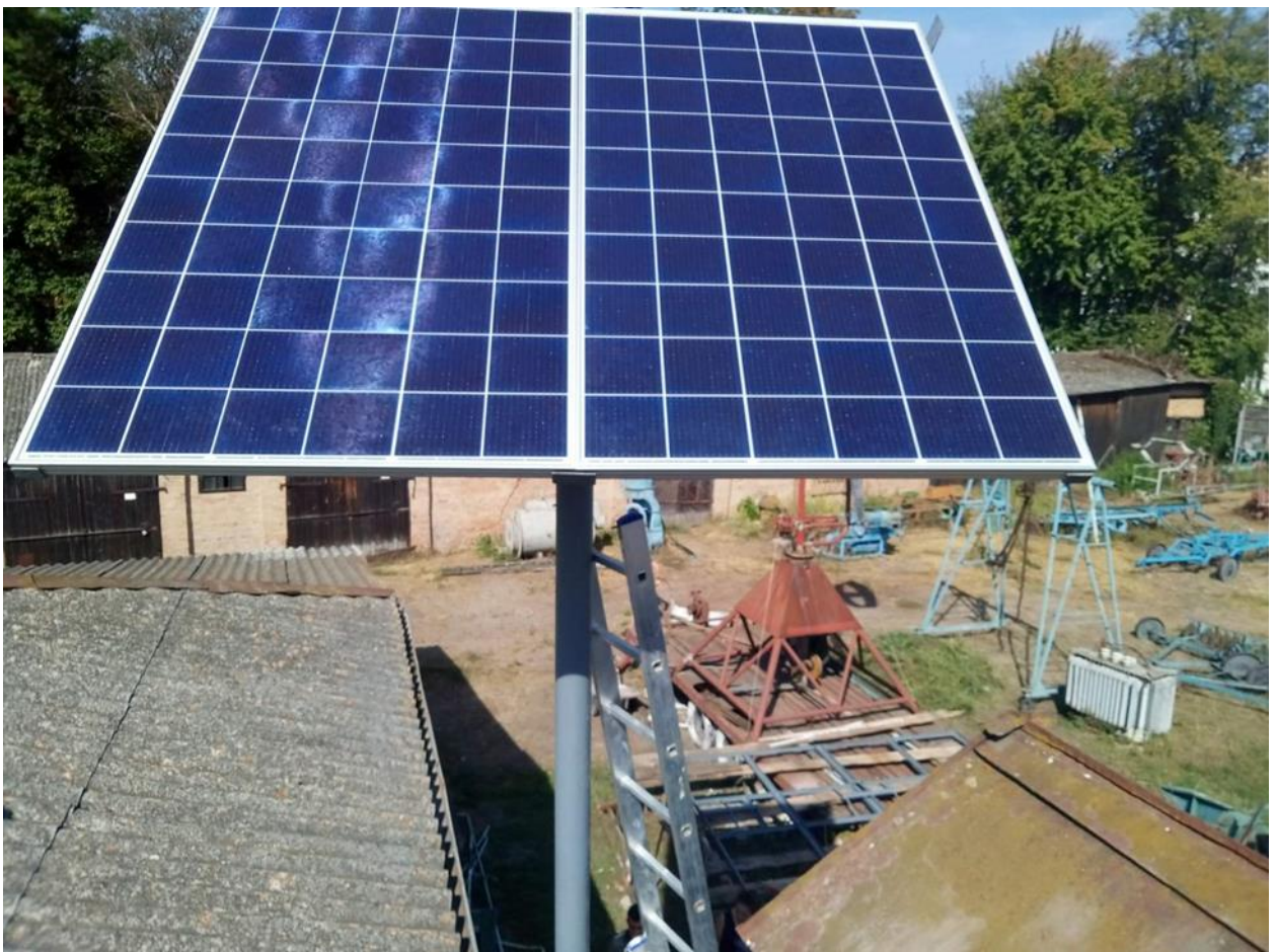
Fig. 1. Photovoltaic panels on a two-axis tracker
